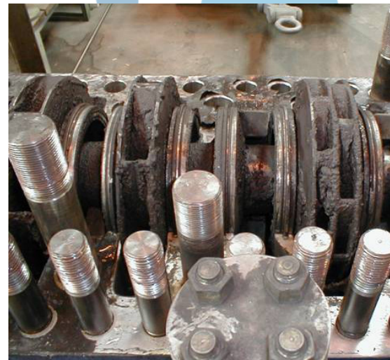
Erosion/scaling of pump parts
